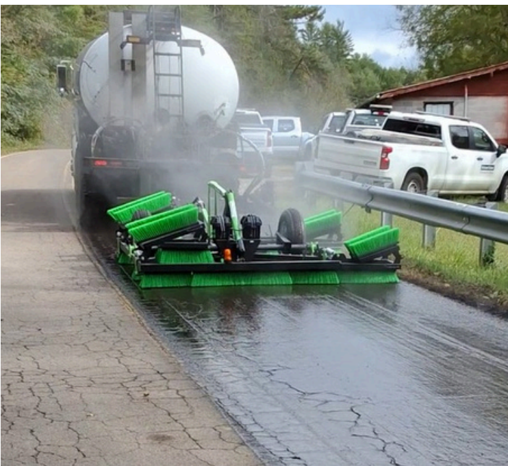
Pictured Below: Scrub Seal paving in Buncombe County.
