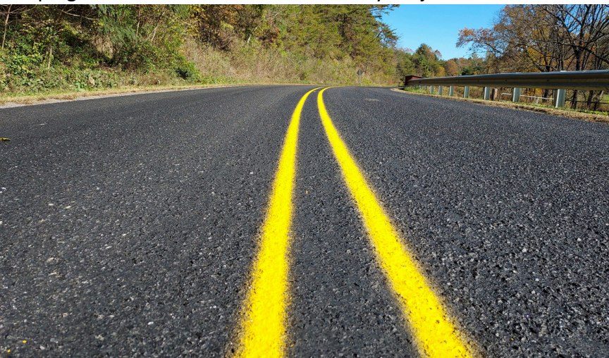
Pictured Above: Aggregate being applied to Scrub Seal emulsion to complete the Chip Seal in Buncombe County.
