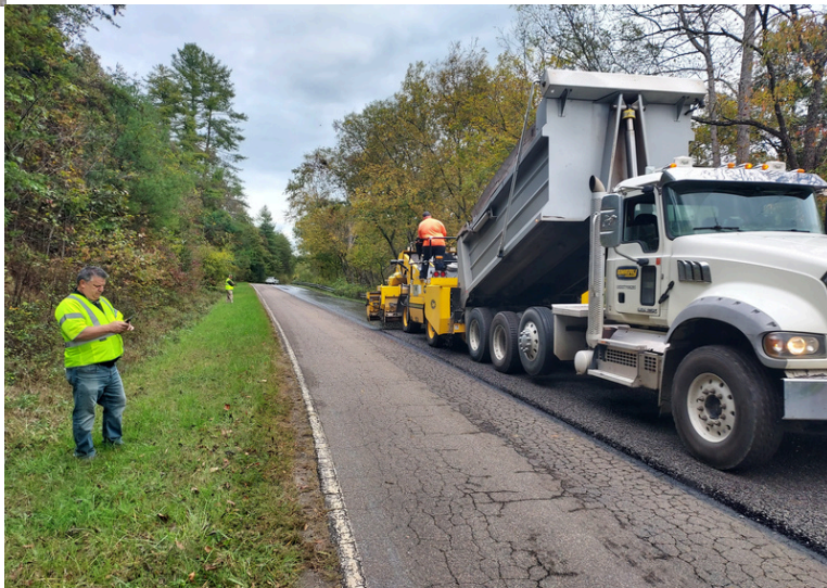
Pictured Above: Aggregate being applied to Scrub Seal emulsion to complete the Chip Seal in Buncombe County.
